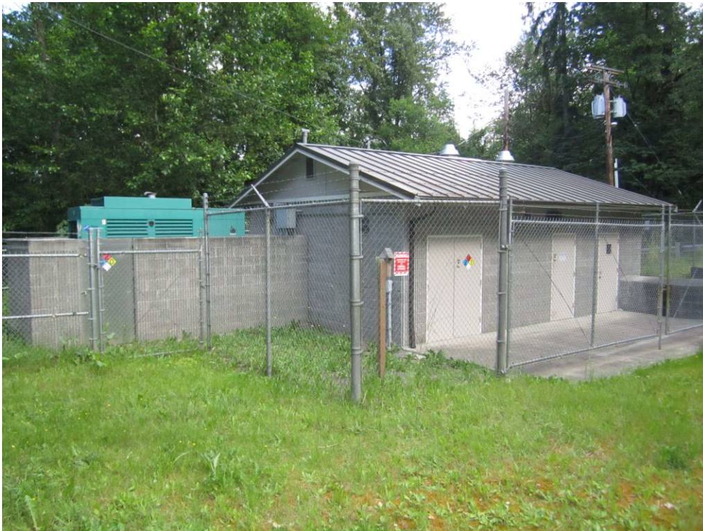
Victor Falls Pump Station
